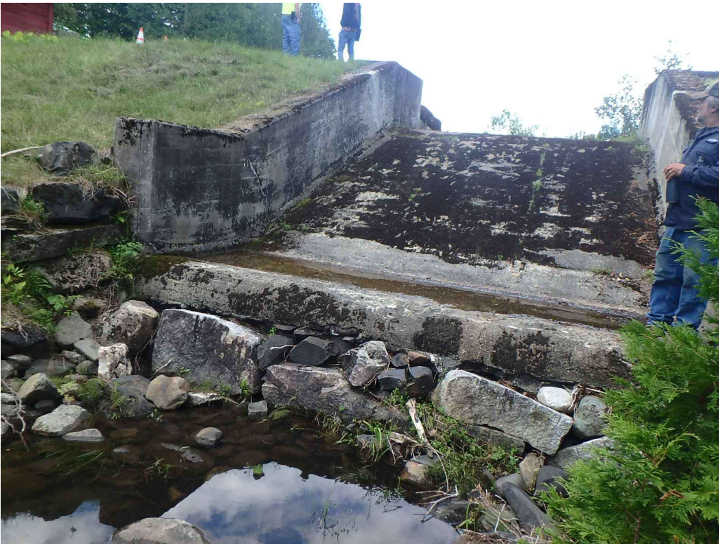
Photo 6: Water pooled below base of auxiliary spillway.
