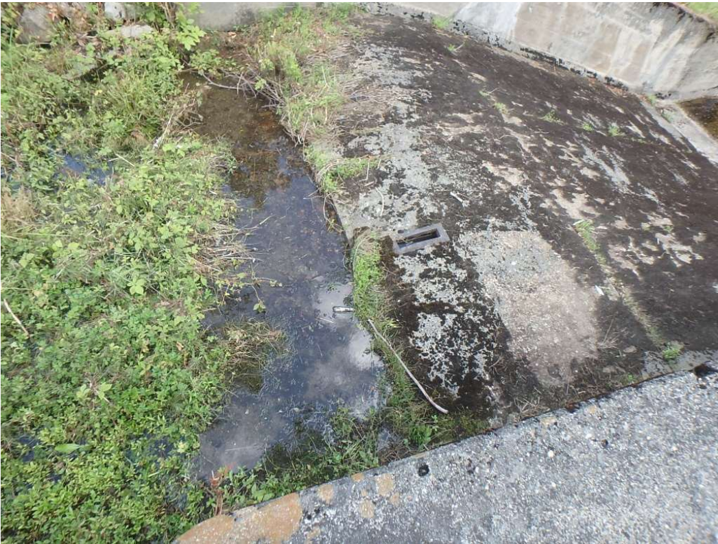
Photo 6: Water pooled below base of auxiliary spillway.
